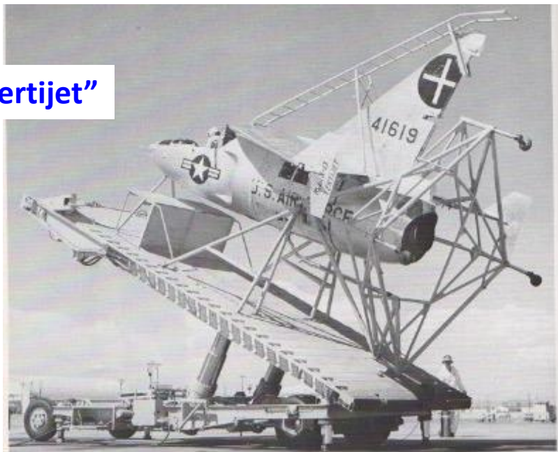
Shown at Grando AFB, first X-14 appears entire jet in vertical support bracket. These were built purely for vertical "Vertijet" VTOL, not all was the original folder which spanning from the vertical line up to the cockpit. Note massive hydraulic rams for lifting. Water-filled to vertical position. Maxine Wagner, Translucence flyer.
